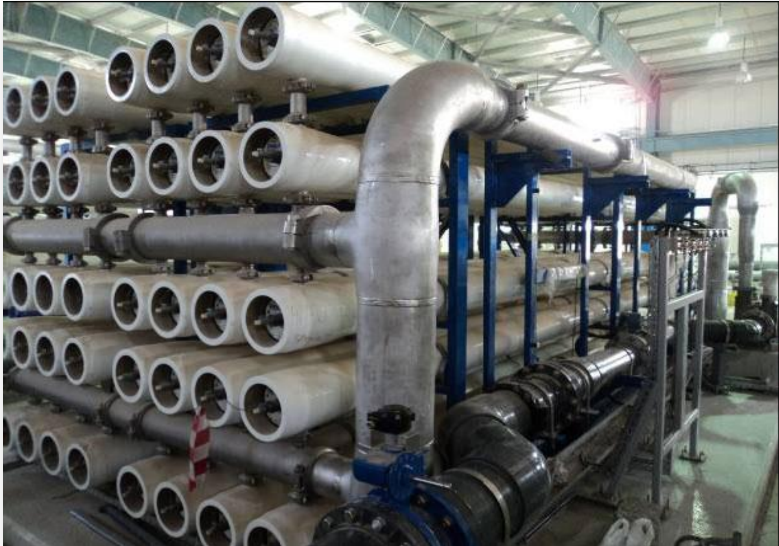
1 st PASS RO – DELMA ISLAND AT ABU DHABI - 3.3 USMGD Pass 2 completed 2012
